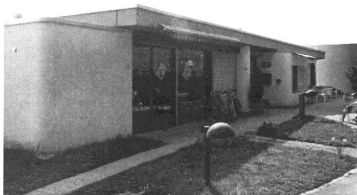
Reinacherstrasse 66, Münchenstein Tennis-Center
