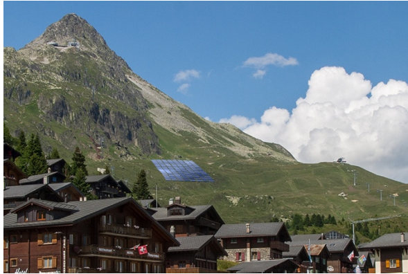
Level 1: Conventional PV panels
